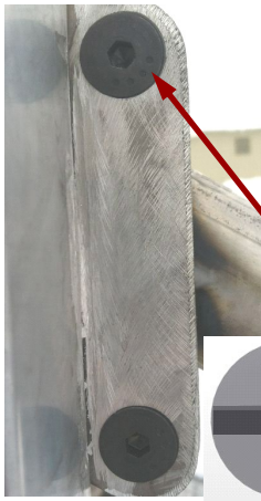
Welded connection plate on columns and U-tube
