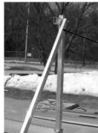
Diagonal Support Tube 2" x 3" x 82 1/4"
