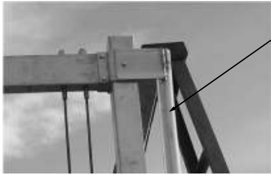
Column Kitty Corner View
