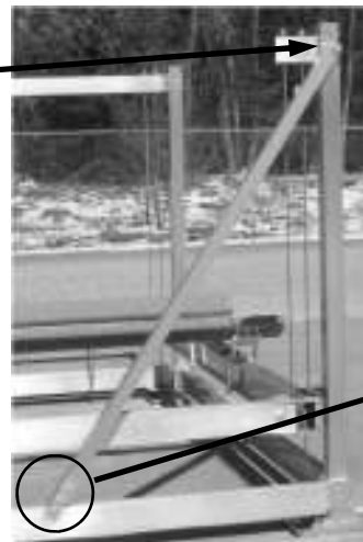
View of 3/16 x 3 x 6" long flat bar (4-req'd) on diagonal braces secured with 3/8 x 2 3/4 bolts and 3/8 whiz nuts. (6-req'd)
