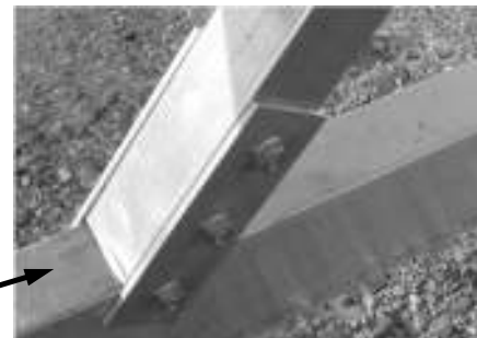
View of 3/16 x 3 x 6" long flat bar (4-req'd) on diagonal braces secured with 3/8 x 2 3/4 bolts and 3/8 whiz nuts. (6-req'd)
