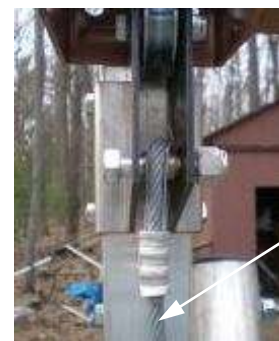
Cable from lift beam`
