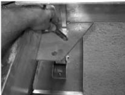
Next take the short cable fitting coming out of the bottom of the twin beam on winch column side of hoist and put it through the nearest hole to column. Put a 5/8" nylon insert lock nut on the back side and tighten so some threads are sticking out from the nut. Use a wrench on the cable machined flats to turn nut. Repeat on other end.
