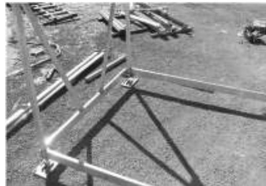
Before tightening bolts, square (tram) the corners of the hoist with equal measurements see next page for example photo.
