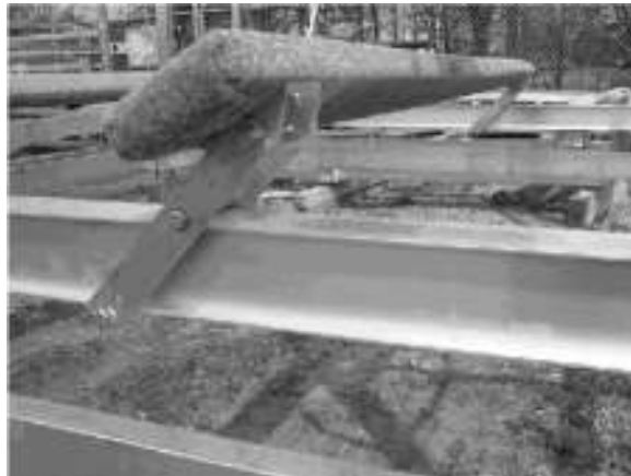
Bunks shown assembled on the hoist. Fit and adjust to boat. Boat weight should be loaded 100% on the bunks.
