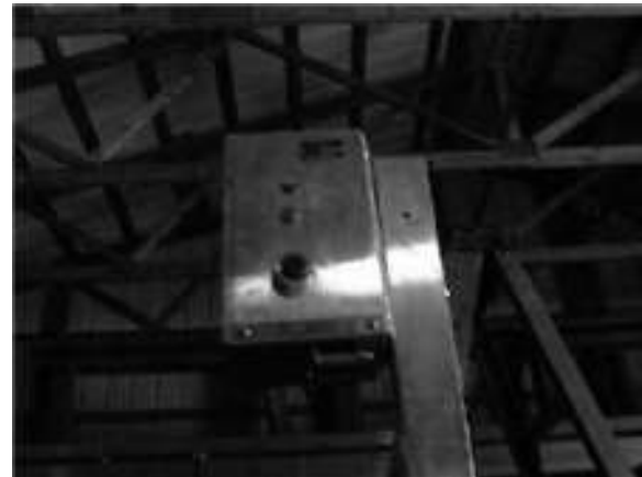
View of winch on column.
