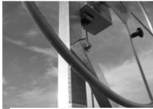
View of winch end with diagonal support
