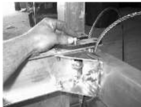
Non winch front side of hoist. Placing guide plate on
