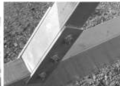
View of 1/4 x 2 x 6" long flat bar (4-req'd) on diagonal braces secured with 3/8 x 2 3/4 hex bolts and 3/8 whiz nuts. (6-req'd)
