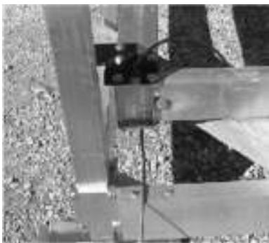
View of winch column area
