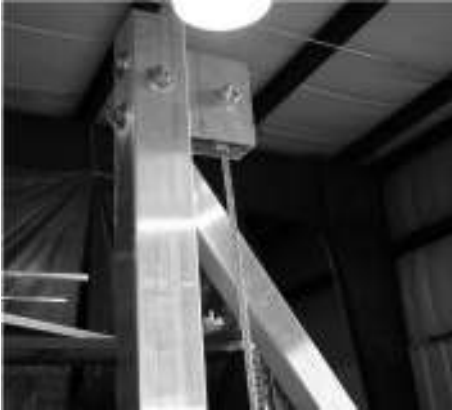
View of winch side, rear corner of hoist. Viewed from inside of the hoist.
