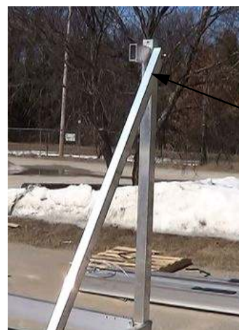
Diagonal Support Connection on Winch Column Opposite
