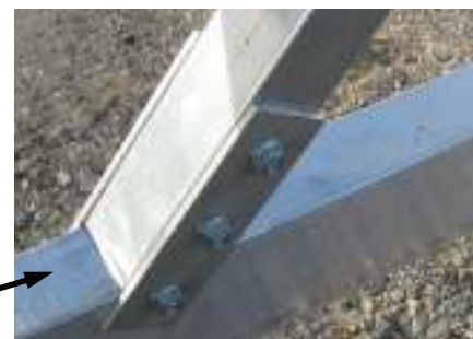
View of 3/16 x 2 x 6" long flat bar (4-req'd) on diagonal braces secured with 3/8 x 2 3/4 hex bolts and 3/8 whiz nuts. (6-req'd)
