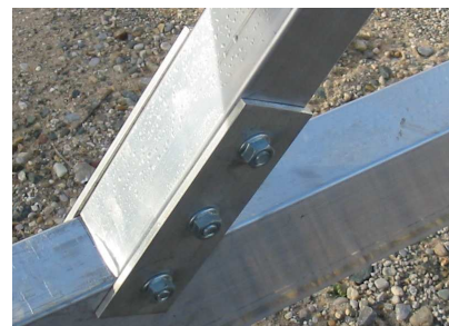
View of 1/4 x 3 x 6" long flat bar (4-req'd) on diagonal braces secured with 3/8 x 2 3/4 hex bolts and 3/8 whiz nuts. (6-req'd)
