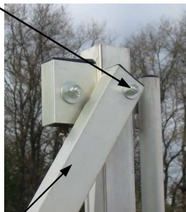
Close up of rear column brace connection
